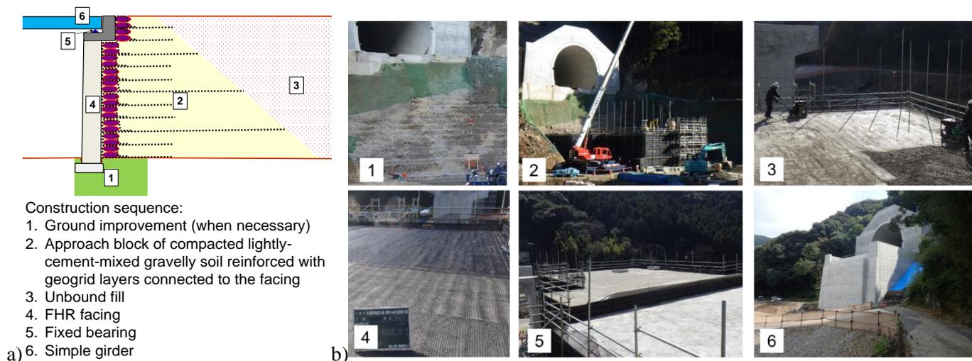
Figure 22. GRS Bridge Abutment (second generation): a) structure and construction procedure; and b) views during construction on a slope at Sugamuta viaduct, Nishi-Kyushu Route, Kyushu Shin-kan-sen (High Speed Railway) (Soga et al., 2018).
