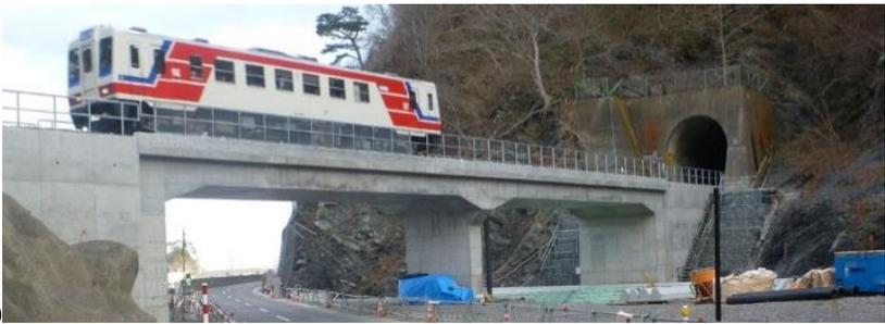
Figure 30. GRS Integral Bridge at Koikorobe, Sanriku Railway (the continuous girder is vertically supported by a central pier): a) structure; and b) April 2014 (Tatsuoka et al., 2015, 2016; Tatsuoka & Watanabe, 2015).
