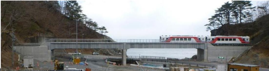
Figure 29. GRS Integral Bridge at Haipe, Sanriku Railway (the continuous girder is vertically supported by a central pier): a) structure; and b) April 2014 (Tatsuoka et al., 2015, 2016; Tatsuoka & Watanabe, 2015).
