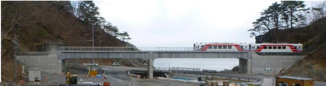
Figure 29. GRS Integral Bridge at Haipe, Sanriku Railway (the continuous girder is vertically supported by a central pier): a) structure; and b) April 2014 (Tatsuoka et al., 2015, 2016; Tatsuoka & Watanabe, 2015).
